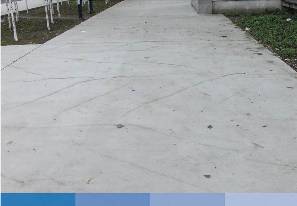
Random shrinkage cracks due to insufficient protection of fresh concrete
