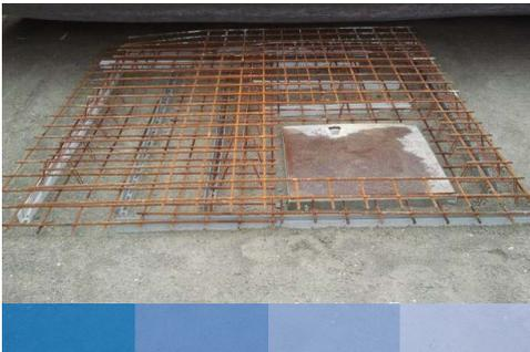
When meshes are combined with dowels, it is important that the meshes overlap the free ends of the dowels. The meshes can be interrupted or cross the joint. In the latter case, they must be sawn above the section of the dowels as described above, as they must themselves remain intact.
