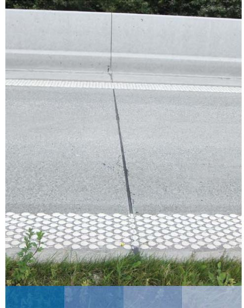
Sympathy cracks initiated by a joint in an adjacent slab or water gutter
