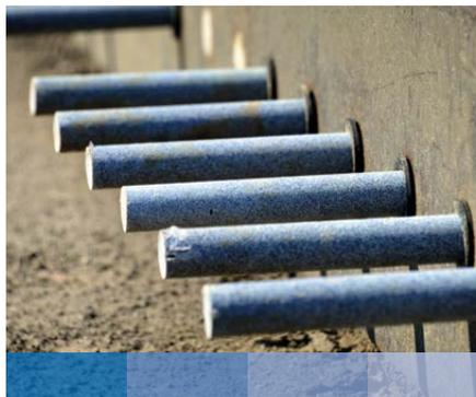
In the case of unbound base layers, the fresh concrete can be dumped with a crane on the next row of dowels, so that they no longer can be displaced during the passing of the slipform paver. Dowel baskets can also be fixed with metal stakes or anchor pins in the unbound aggregate base.
