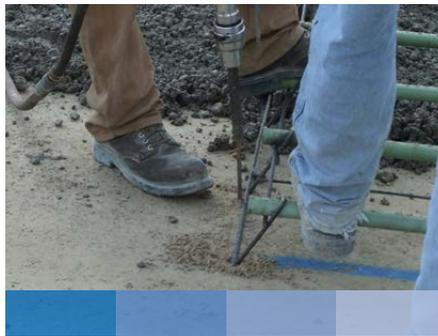
Automatic insertion of dowels in the fresh concrete (photo: Betonhuis, NL)
