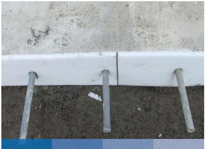
Another important issue is the size of the filler. Its length must be equivalent to the width of the pavement. If this is not the case, compressive stress concentration at the ends
