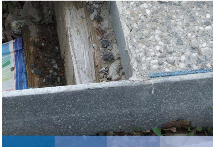
Recycled T-shaped PVC used as a construction and contraction joint
