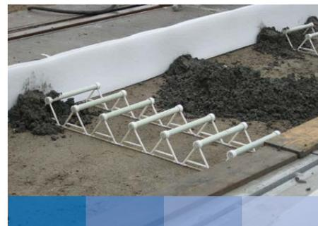
Plate dowels installed in a construction joint (photo: Danley, U.K.)
