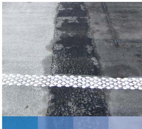
Shortened anchoring abutment for transition between concrete and asphalt
