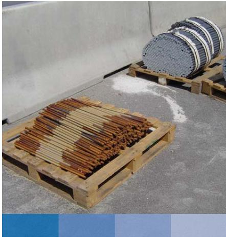
The tie bars are placed at mid-depth of the pavement, perpendicular to the driving direction, spaced and at a distance from the transverse joint of about 750 mm to 1000 mm.
