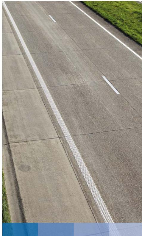
Example of correctly positioned longitudinal joints and road marking (photo: A. Nullens for FEBELCEM)
