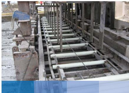
The dowels are specified in the European standard EN 13877-3 entitled "Concrete pavements - Part 3: Specifications for dowels to be used in concrete pavements". The minimum tensile strength required is 250 MPa and the durability must be declared by the manufacturer. It is also
