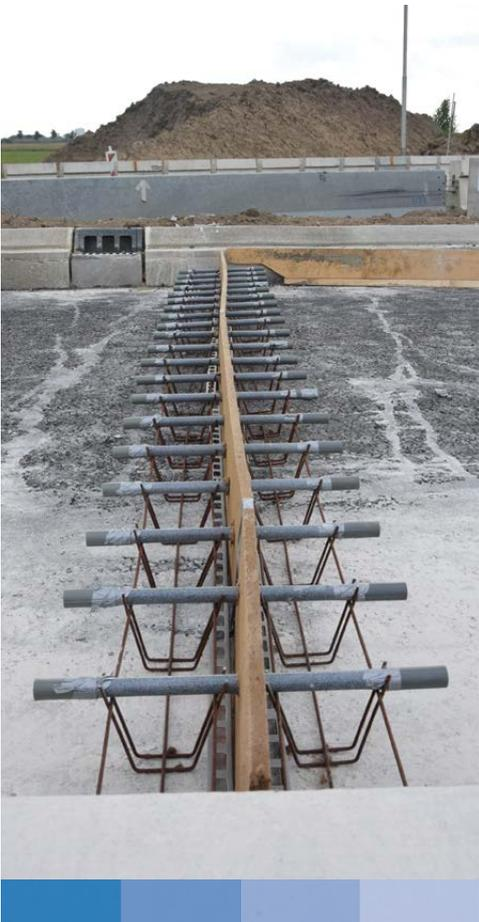
Sawed cutout, allowing positioning the filler of the expansion joint
