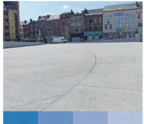
Charleroi, Place de la Digue: to avoid sympathy cracks in this staggered joint layout, isolation membranes were placed along the longitudinal joints
