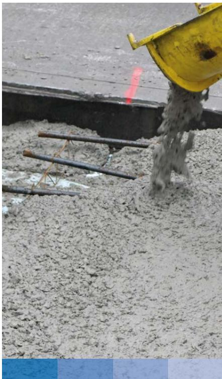
Dowel baskets fixed on an asphalt sandwich layer (top) and glued in a construction joint (bottom – photo: BKB-Infra)
