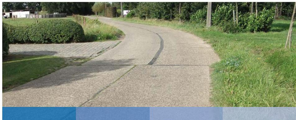
Also free-movement longitudinal joints can be considered, using tapered plate dowels, working in conjunction with free-movement contraction joints.
