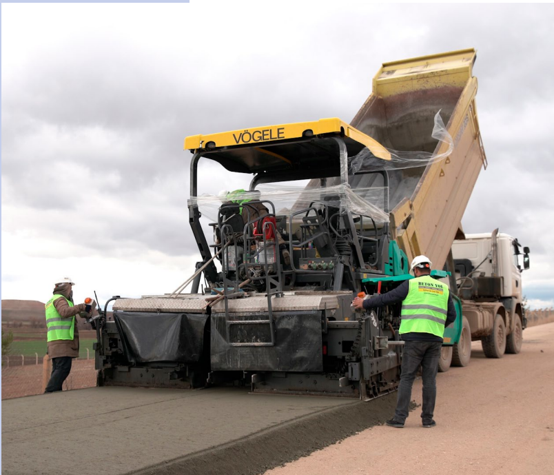
Construction of a RCC road - Photo: Türkcimento
