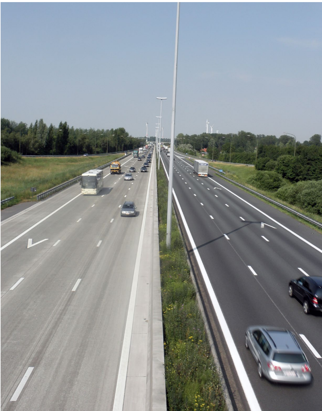
Motorway in concrete and asphalt - Photo: Luc Rens
