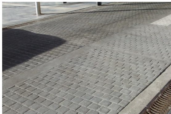
Cobblestone pattern – using moulds
