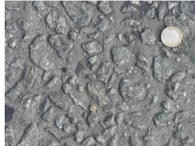
Rolling noise for an EAC surface due to (too) large coarse aggregates in the concrete mixture
