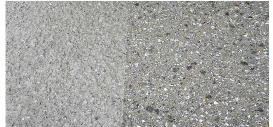
Surface before and after HDW
