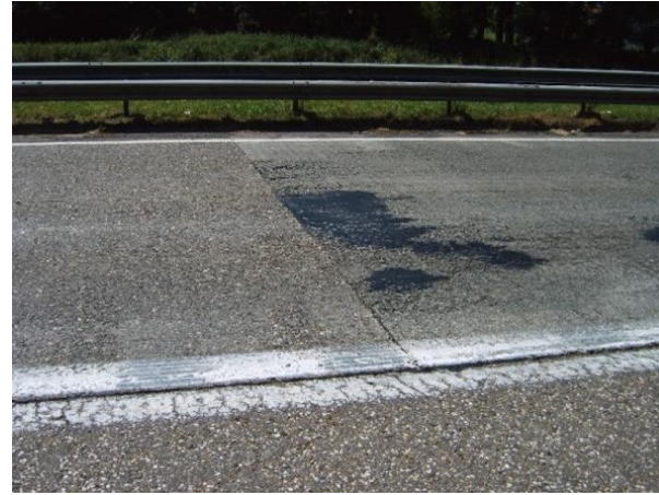
Transverse construction joint in CRCP, with increased risk of water penetration
