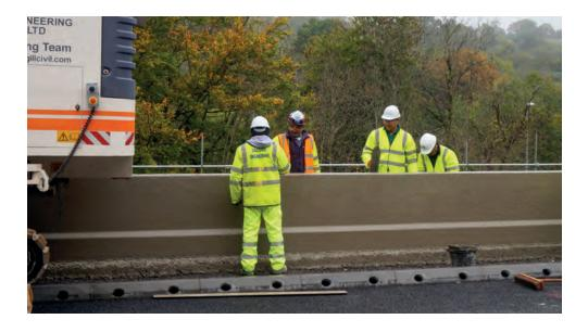
Concrete barriers may be surface mounted or embedded with foundations. Surface mounted offers particular benefits of reduced construction times and reduced costs. In addition to speed of construction, slipformed concrete barriers offer a finish without joints, reduced labour costs, long-term performance and minimum maintenance.
