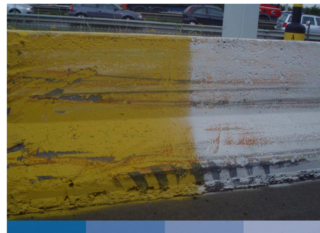
Traces of tyres on a concrete safety barrier, showing its resistance to vehicle impacts
