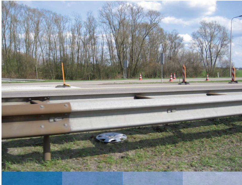
Example of corrosion of a steel guardrail
