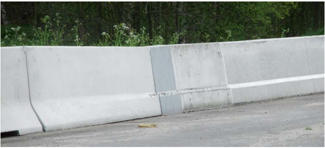
Transition between a concrete step barrier and a steel system
