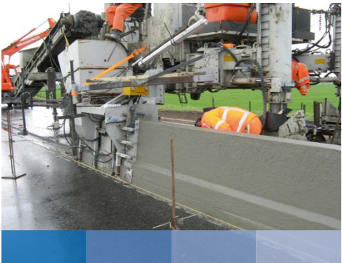
Surface mounted CSB installation
