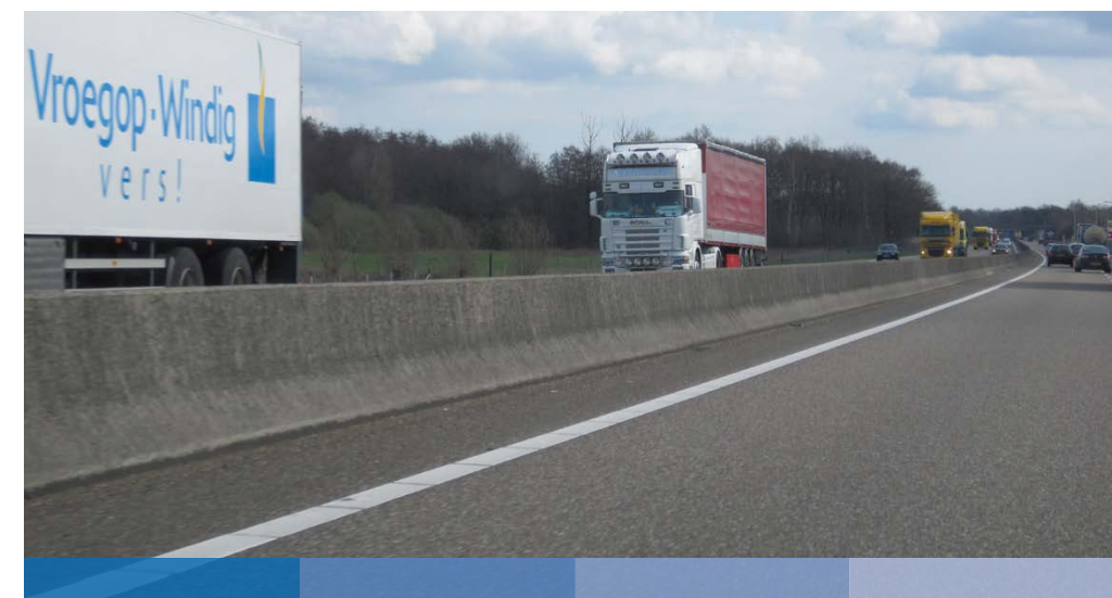
New Jersey barrier in the central reserve of a motorway
