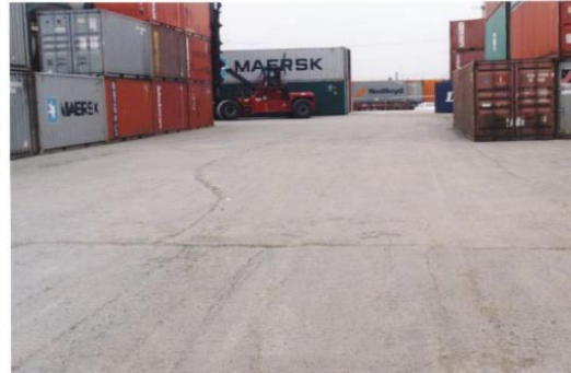
Conley Terminal, Boston, MA (built 1986)
