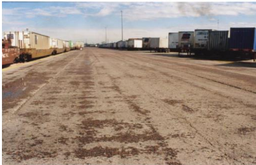
Intermodal Terminal, Denver, CO (built 1986)
