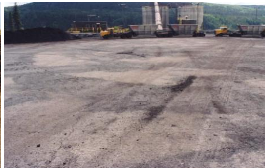
Storage of coal, Vancouver, B.C. (built 1992)
