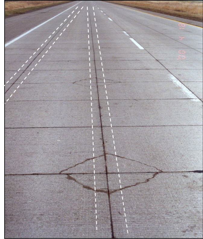
1.2m x 1.2m Panels: Corner Breaks due to Wheel Loadings
