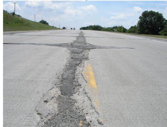
Missouri county road, pre-overlay condition, no repairs prior to 125mm unbonded overlay (2008)
