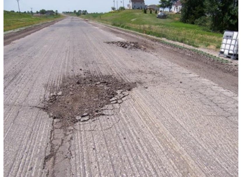
Excessive milling of existing asphalt
