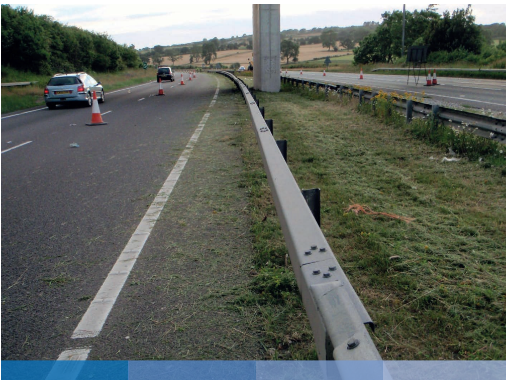
Figure 4 Open Box Beams protecting a bridge pier © John Elystan Richards
