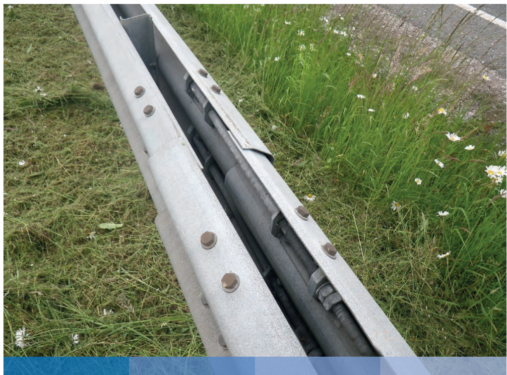
Figure 5 Double Sided TCB with tensioning assembly © John Elystan Richards
