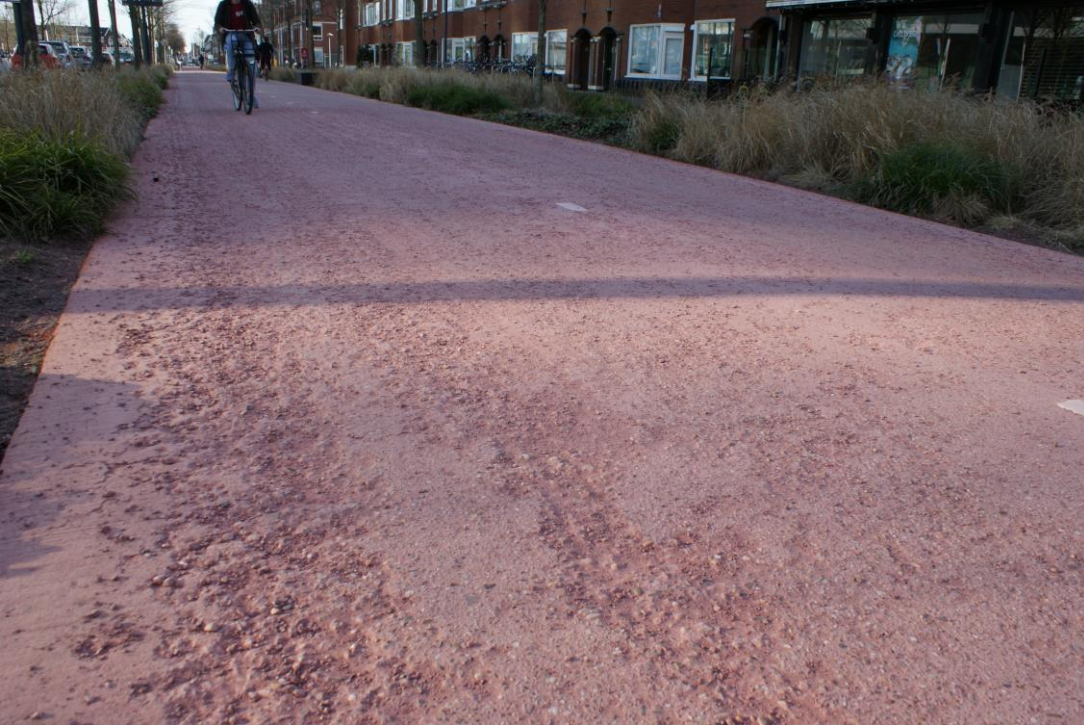
Cycle path (Croeselaan, Utrecht) Construction: spring 2018 Picture: February 2021
