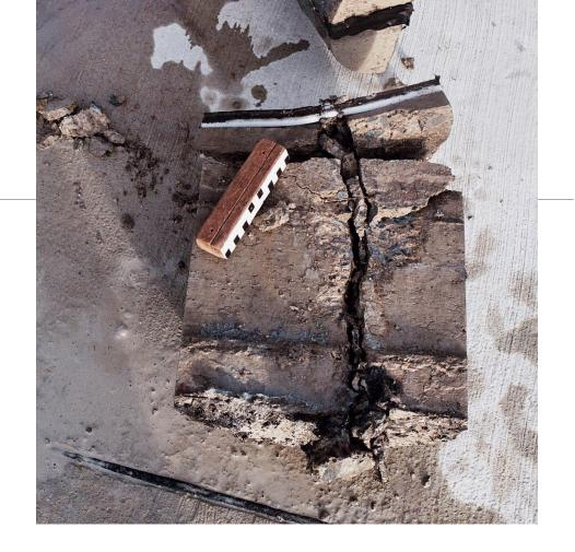
Depth of saw cut: at least 1/3 of total thickness
