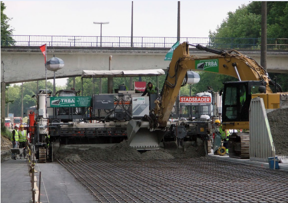
Construction of a CRCP - Photo: Luc Rens
