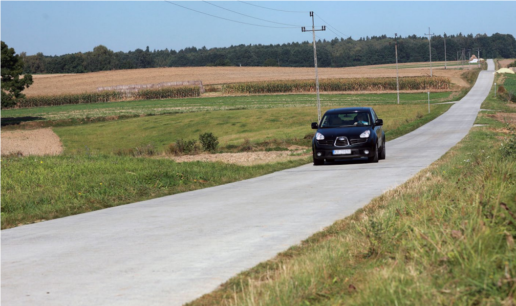
Local road in concrete - Photo: Polish Cement Association
