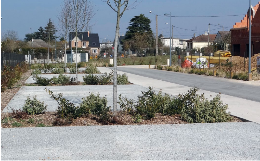
Parking lot in pervious concrete pavement, Dreux (France) © CIMbéton
