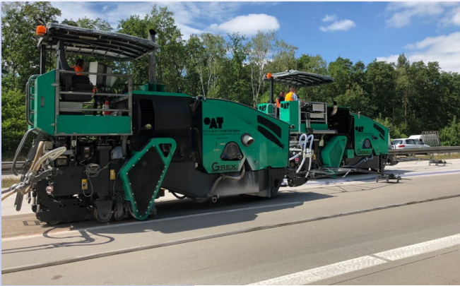
Grinding machine in operation and a finished very low-noise "Next Generation Concrete Surface"
