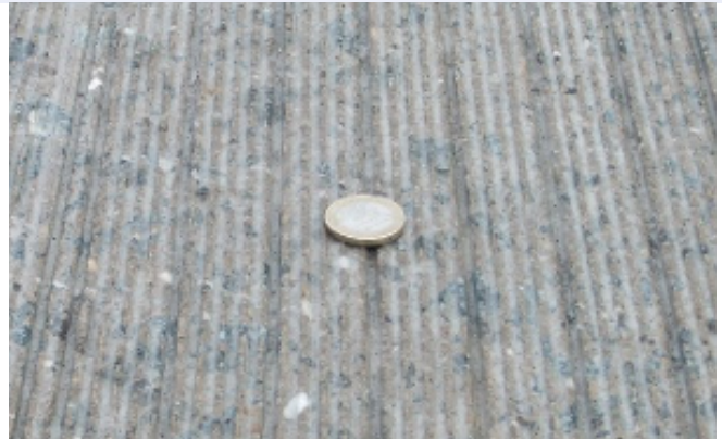
Grinding machine in operation and a finished very low-noise "Next Generation Concrete Surface"
