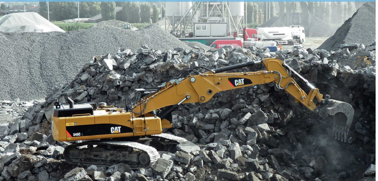
Concrete pavement recycling – motorway E17, De Pinte, Belgium, 2011 © L. Rens / FEBELCEM
