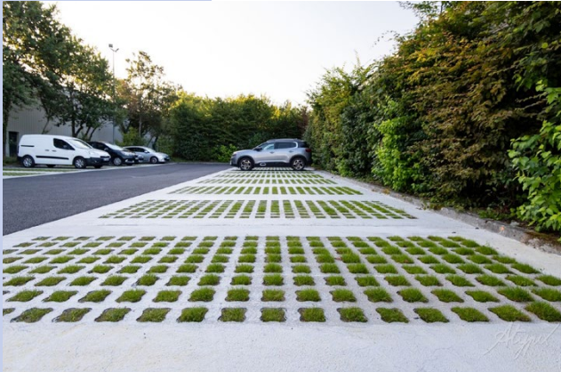
Applications of cellular reinforced concrete for a parking lot and a tramway © Viaverde
