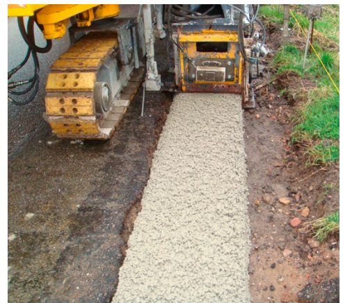
Construction of 'Bermcrete' in the Netherlands © Heijmans
