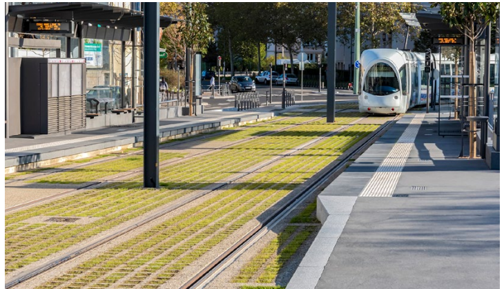
Applications of cellular reinforced concrete for a parking lot and a tramway © Viaverde
