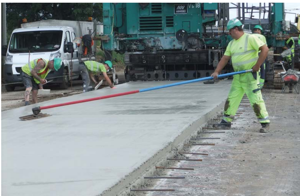
Finishing with a long-handled float
