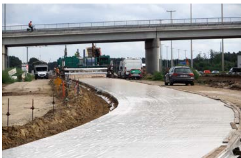
Reduced stake interval in a curve
