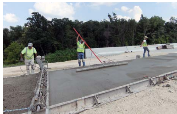
Examples of steel and plastic side forms
