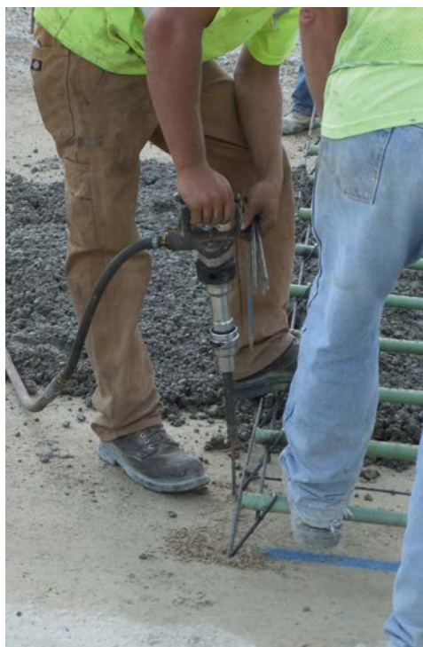
Positioning of dowels: fastening of the dowel basket –placing concrete upon the dowel assembly
