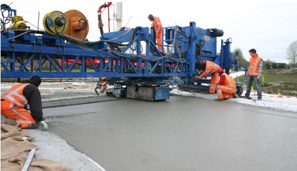
Use of a roller finisher for the construction of a concrete roundabout (Photo: Cement&BetonCentrum)
