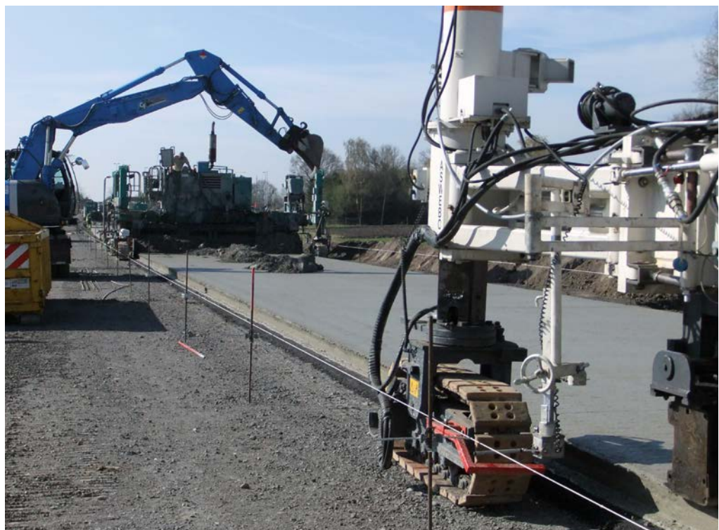
Two-layer paving operation
