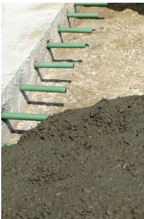
Doweled construction joint
