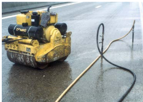
Injection of the grout
