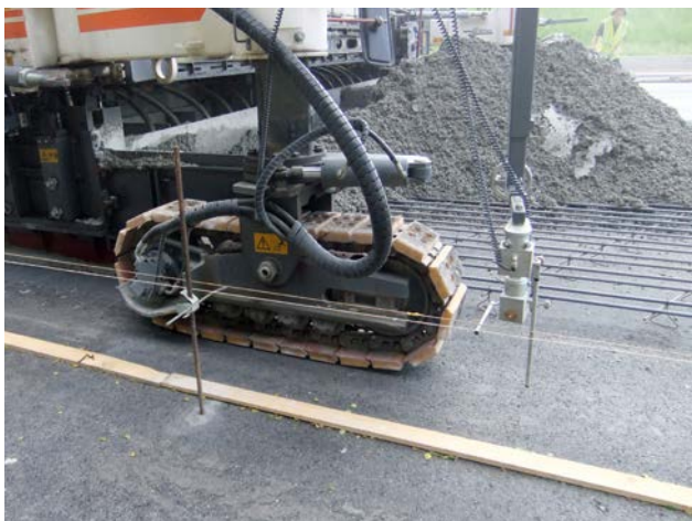
Rolling path for slipform machine; left picture: on an asphalt interlayer; right picture: on a widened subbase layer
