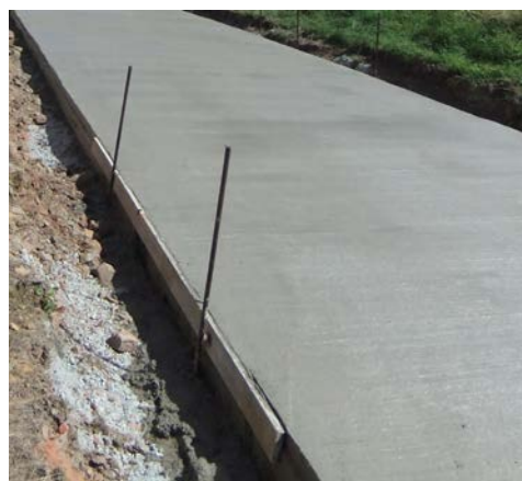
Local repair of an edge failure
