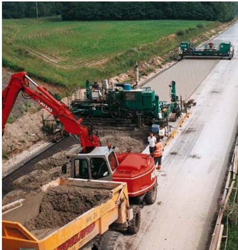
General view and close up of a slipform paver using an averaging ski
