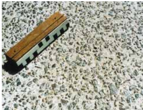
Texture of an exposed aggregate concrete 0/14 (Brussels, Lorrainedreef, 2003)
