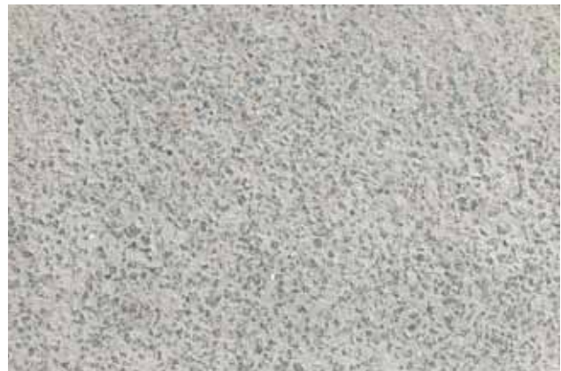
E17 De Pinte – Kruishoutem: single-layer exposed-aggregate concrete 0/20. Noise levels measured with CPX at 80 km/h: 98.5 dB(A) for a truck tyre and 99.1 dB(A) for a passenger car tyre
