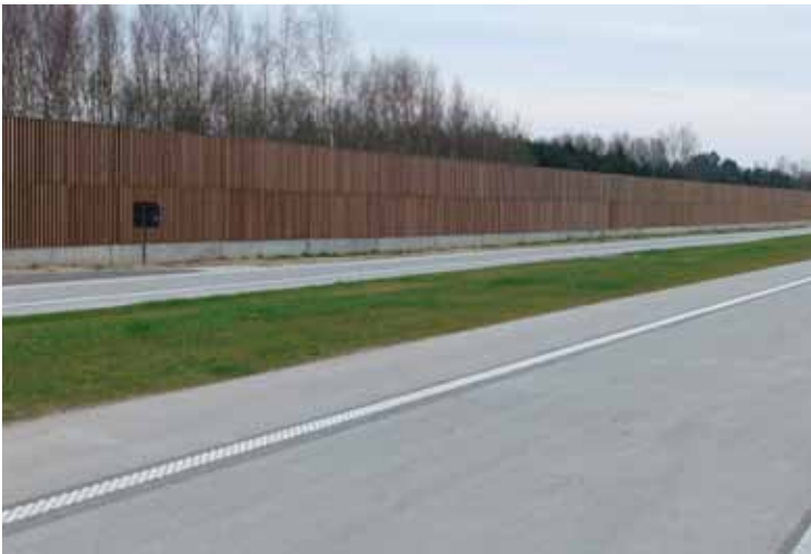
Low-noise double layered concrete pavement combined with noise barriers on the new road link in N19g Geel-Kasterlee (Belgium), realized as a PPP-project.
