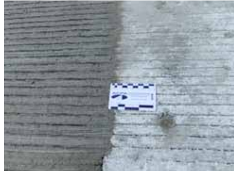
Longitudinal tining of fresh concrete in Illinois, U.S.
