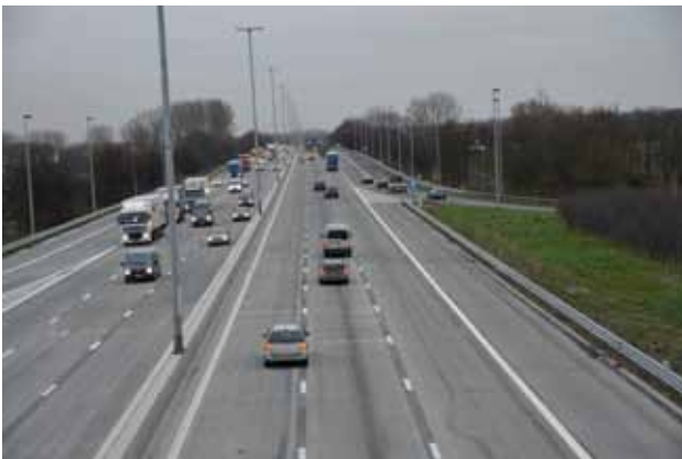
E17 De Pinte – Kruishoutem: single-layer exposed-aggregate concrete 0/20. Noise levels measured with CPX at 80 km/h: 98.5 dB(A) for a truck tyre and 99.1 dB(A) for a passenger car tyre
