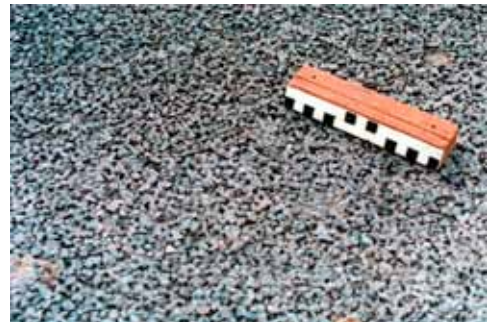
Texture of very open concrete (Herne, N255, 1996)
