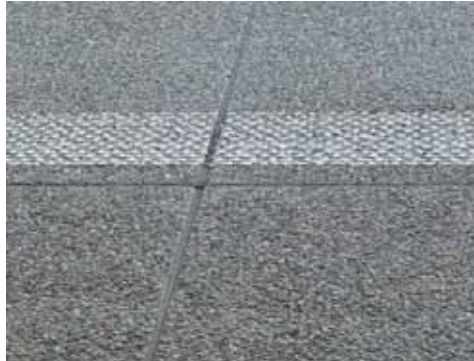
Texture of an exposed aggregate concrete 0/14 (Brussels, Lorrainedreef, 2003)
