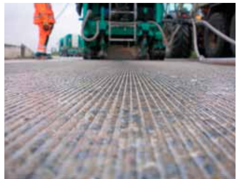
Detail view of the diamond ground surface and texture of the “Geseke access road” in Germany
