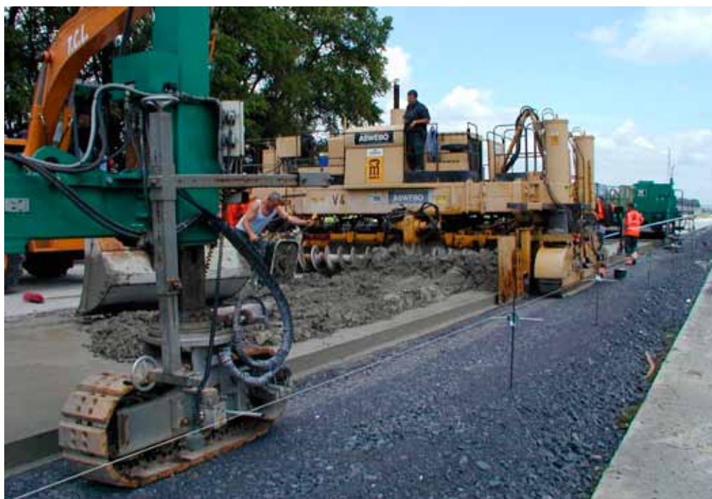
Estaimpuis: construction of the double-layered CRCP
