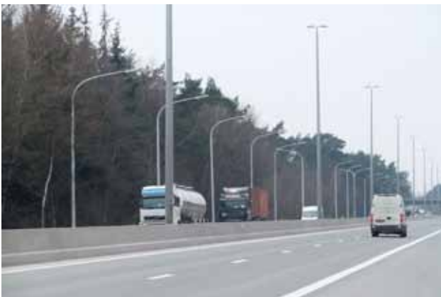
E313 Herentals-Grobbendonk: double-layer exposed-aggregate concrete with top layer 0/6.3. Noise levels measured with CPX act 80 km/h: 98.5 dB(A) for a truck tyre and 98.5 dB(A) for a passenger car tyre
