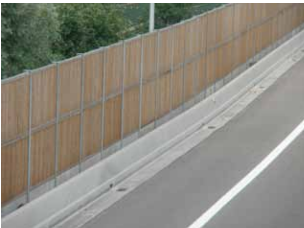
Examples of noise barriers along highways
