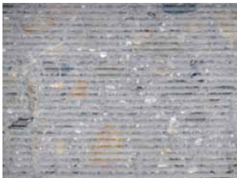
Diamond grinding as restoration technique on old concrete slabs
