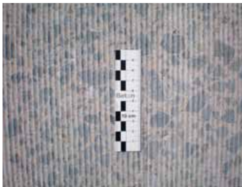
Detail view of the diamond ground surface and texture of the “Geseke access road” in Germany
