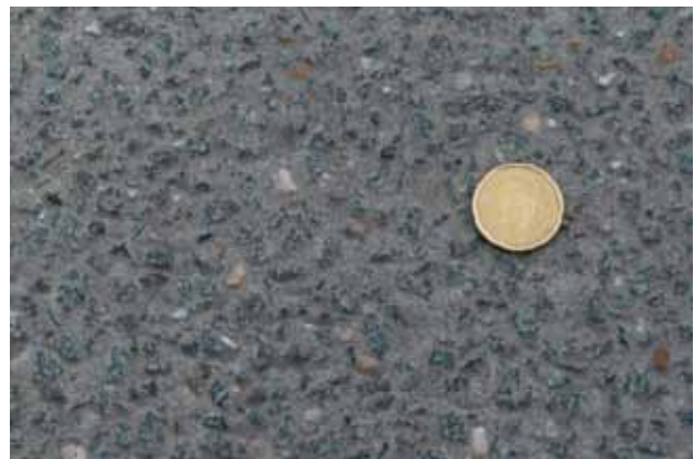
E313 Herentals-Grobbendonk: double-layer exposed-aggregate concrete with top layer 0/6.3. Noise levels measured with CPX act 80 km/h: 98.5 dB(A) for a truck tyre and 98.5 dB(A) for a passenger car tyre
