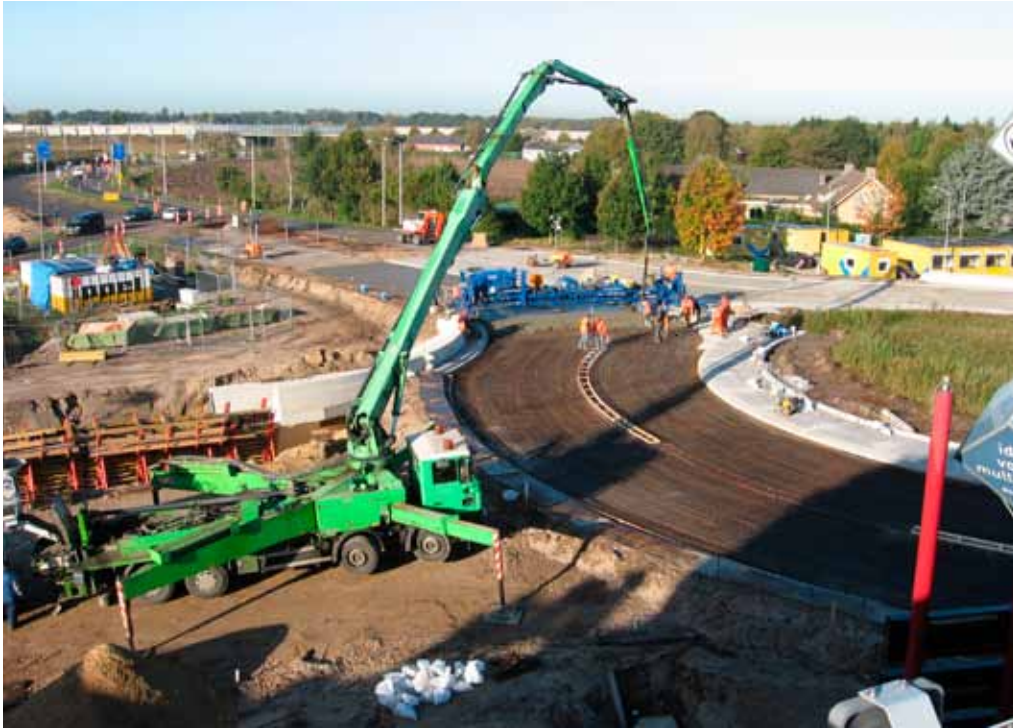
Delivery of concrete by pumping
