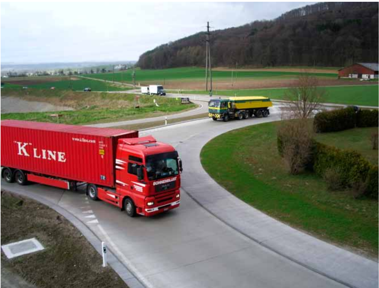
Roundabout in Switzerland (Ref 4)
