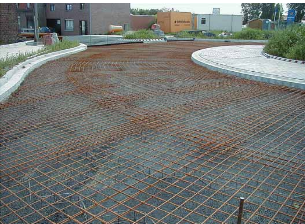
Steel mesh reinforcement (Febelcem)
