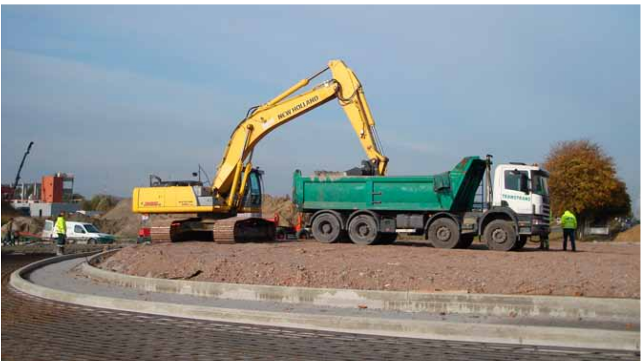
Delivery of concrete from the centre of the roundabout (Ref 2)
