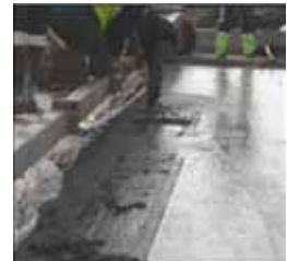
Working over unhardened concrete to complete the roundabout (Ref 2)
