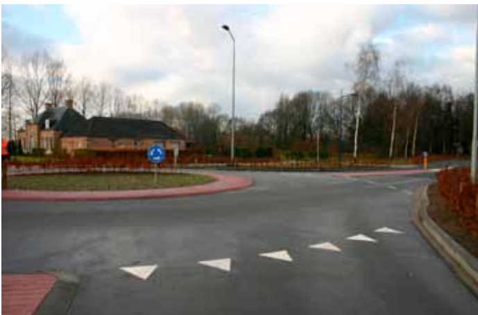
Roundabout in coloured steel fibre reinforced concrete (Ref 1)
