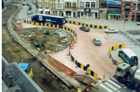
Concreting in 2 separate operations (Ref 2)
