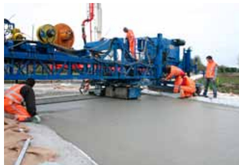
Concreting with a roller-finisher (Photo : W. Kramer)
