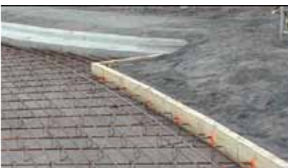
Fixed formwork made of sturdy planks installed on the access roads (Ref 2)
