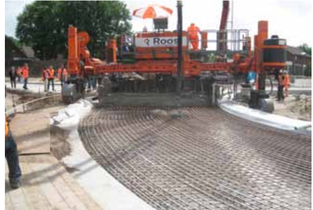
Concreting with a slipform paver (Ref 2 & 3)
