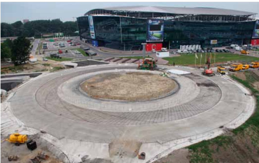
Concreting of different lanes in separate operations (Ref.: Flemish Road and Traffic Agency AWW)
