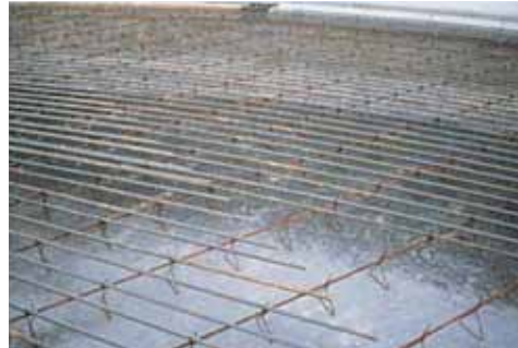
Example of a roundabout in CRCP in Airvault – Deux Sèvres, France (Ref 9)
