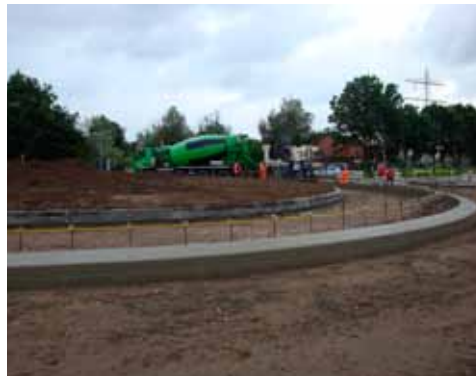
Examples of kerbs cast in-situ in the Netherlands
