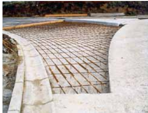
The slabs of the approach legs are reinforced and anchored to the roundabout carriageway (Ref 2)
