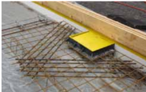
Example of a case where the orange-coloured mark indicates the position of the contraction joint to be cut towards the centre of the manhole (Photo by FEBELCEM)
