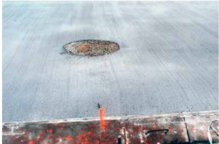
Example of a case where the orange-coloured mark indicates the position of the contraction joint to be cut towards the centre of the manhole (Photo by FEBELCEM)
