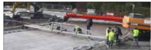
Working over unhardened concrete to complete the roundabout (Ref 2)
