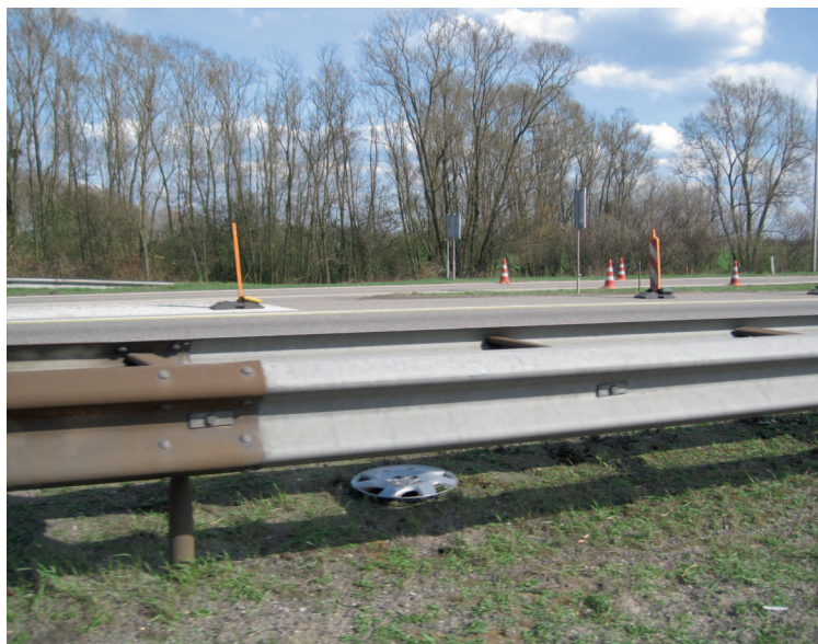
Example of corrosion of a steel guardrail
