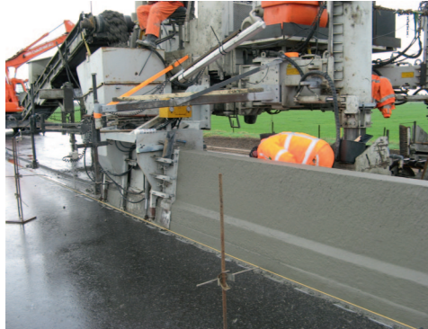
Surface mounted CSB installation
