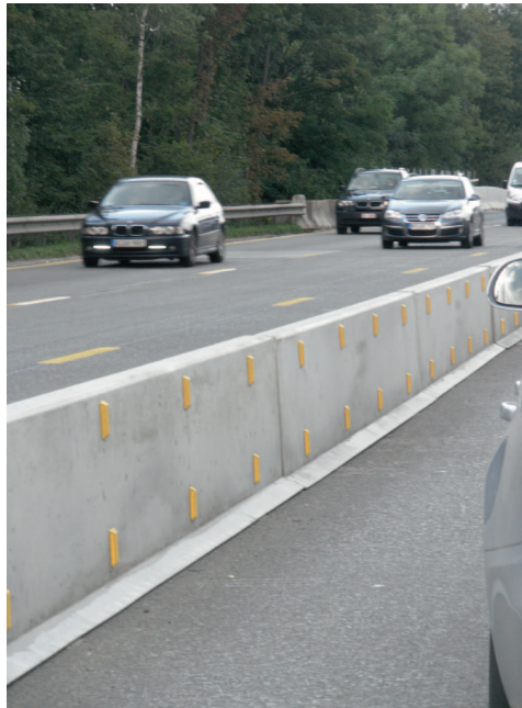
Precast barriers in a permanent and a temporary installation
