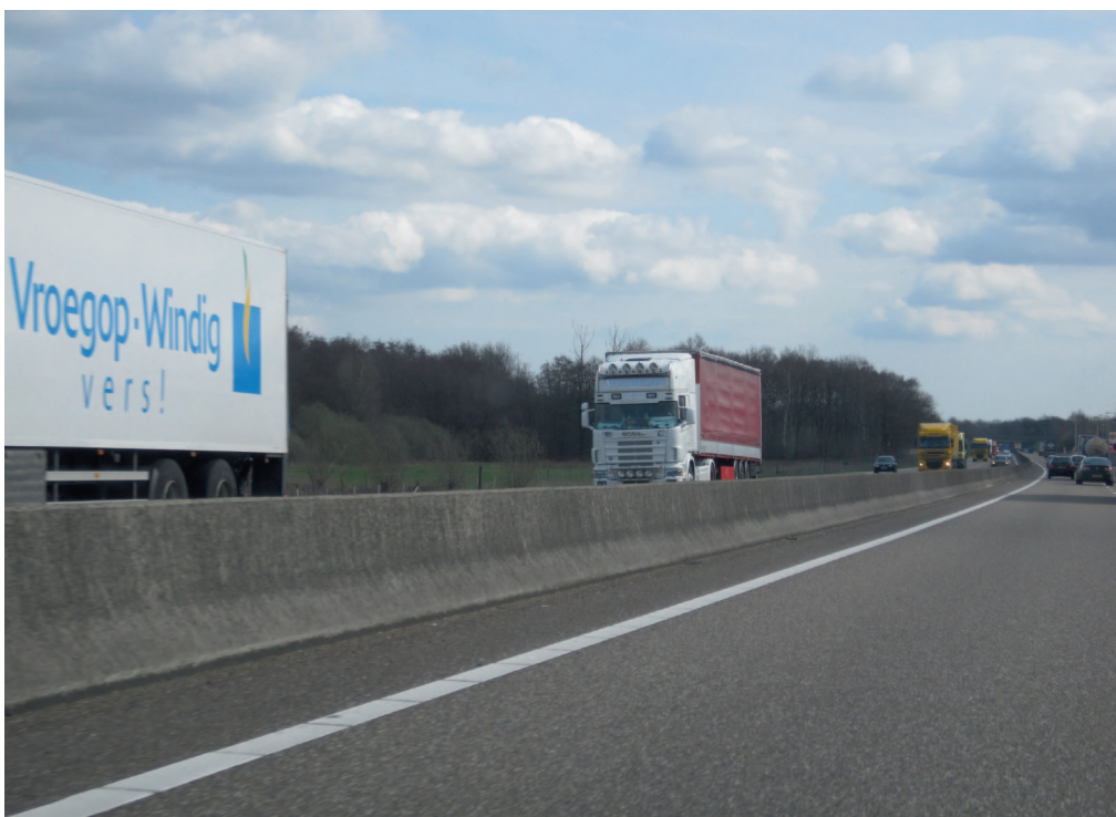
New Jersey barrier in the central reserve of a motorway
