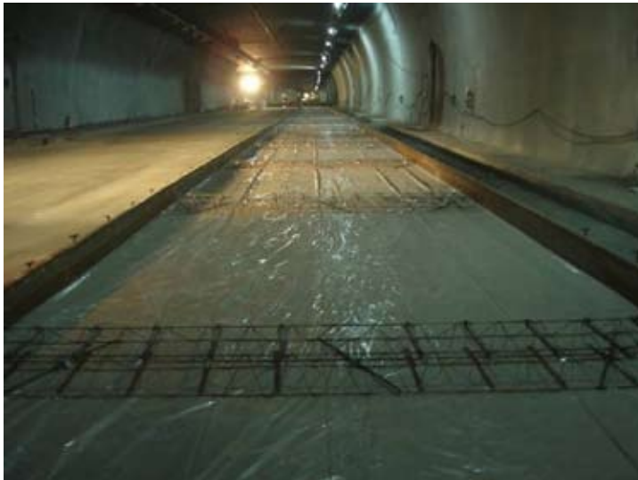
Figure 18: Construction by half widths
