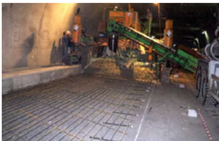
Figure 24: Continuously reinforced concrete pavement constructed by half widths
