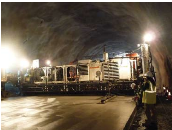
Figure 19: Construction by full width
