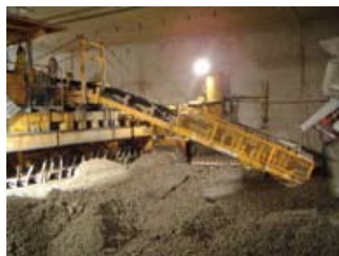
Figure 22: Two layer pavement: supply of concrete of the upper layer
