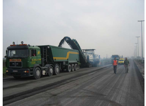
Partly milling off of the asphalt
