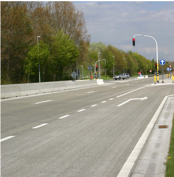
Road widening for a new exit lane in Leuven, Belgium (Ref: L. Rens)
