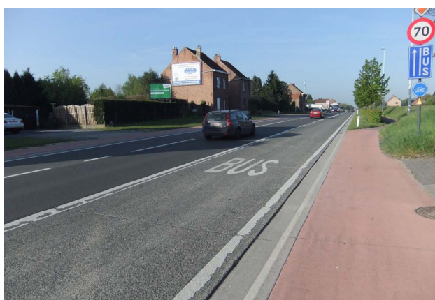
Examples of concrete inlay and road widening for the creation of dedicated buslanes (Ref: Left: L. Rens - Right: A. Nullens)
