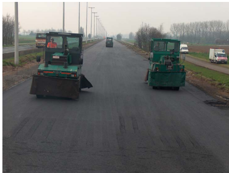
Placing of a new asphalt sandwich layer
