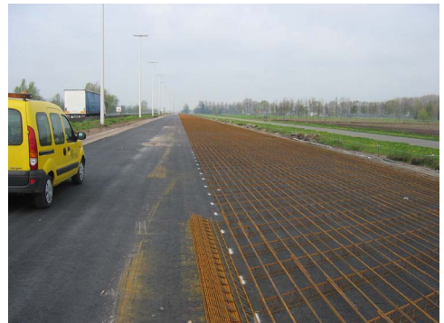
Positioning of steel reinforcement
