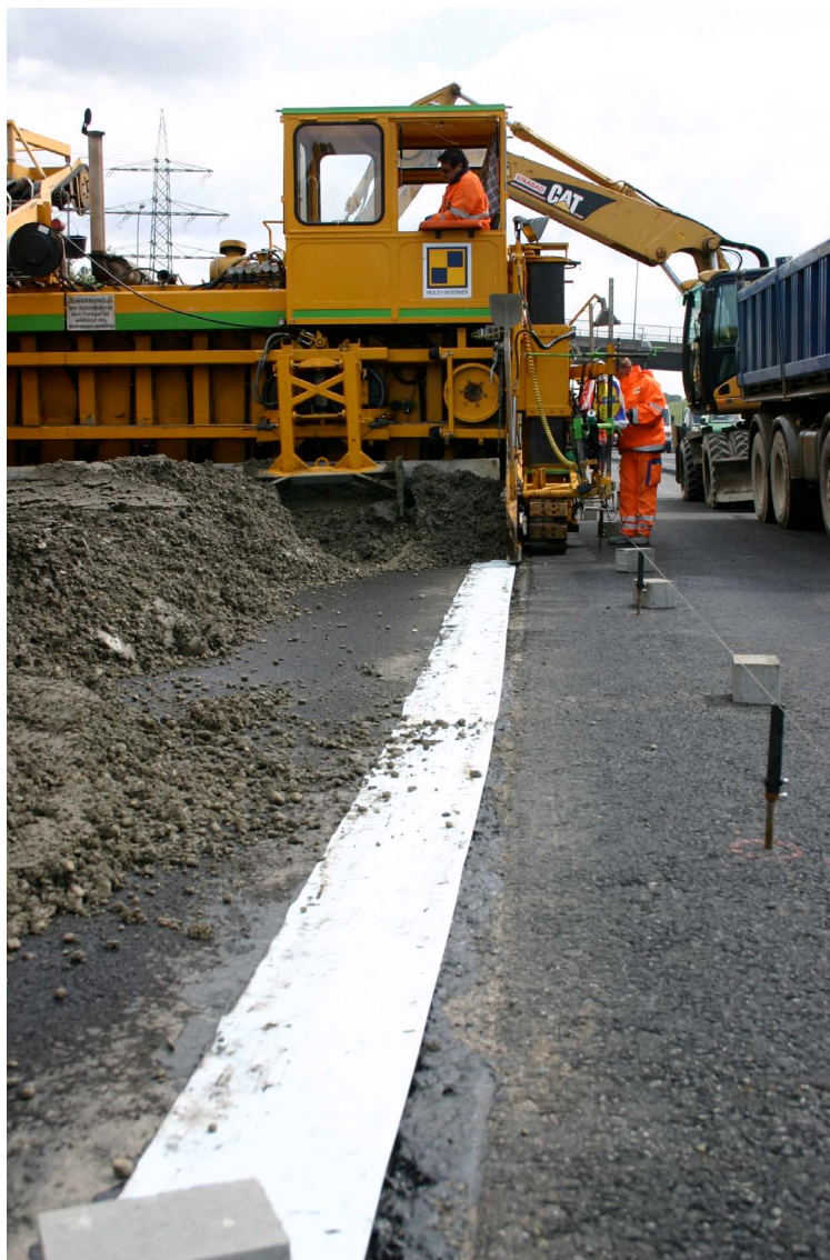
A drain is being constructed to prevent water build-up (Ref: 7 and 9)
