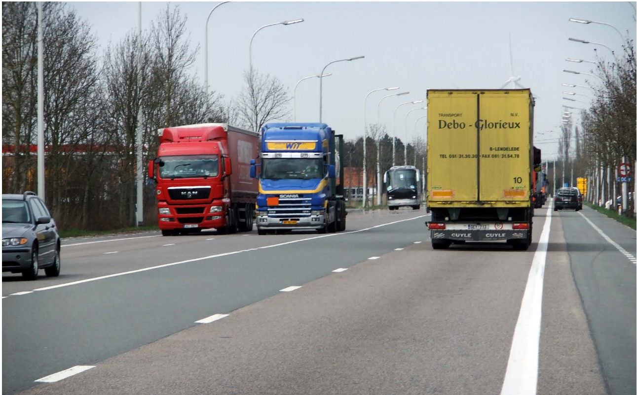
A view of the N31 with the slow lane in concrete and the fast lane in asphalt (Ref: L. Rens)
