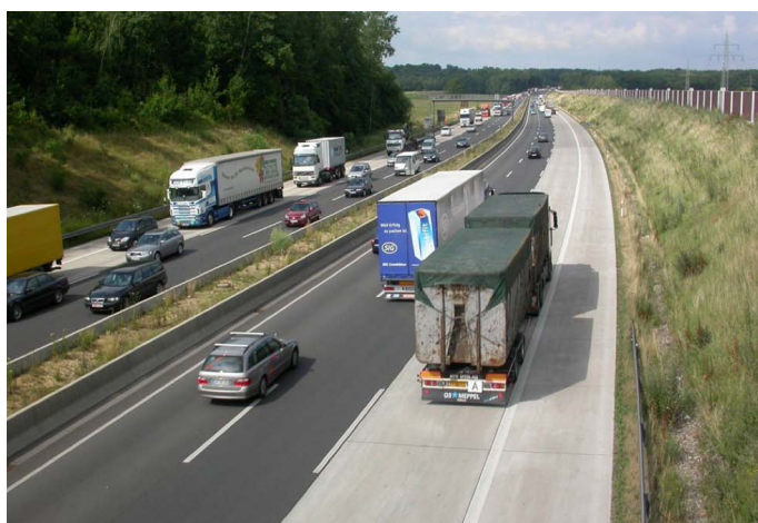
Road widening on motorway A4 in Germany (Ref. 9)
