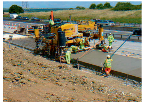
Road widening on the M25 motorway in the UK (Ref: Britpave)
