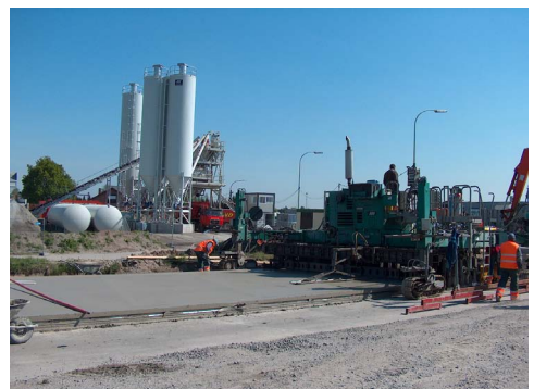
Placing and smoothing of concrete
