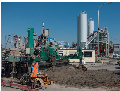
Spreading and compaction of concrete
