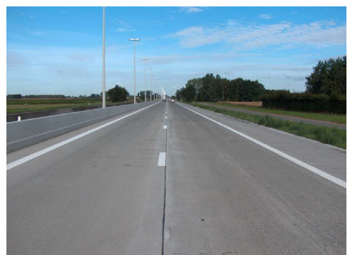
New highway in CRCP
