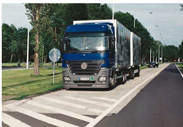
Concrete inlay for a parking strip for heavy trucks (Ref: P. Van Audenhove, CRIC)
