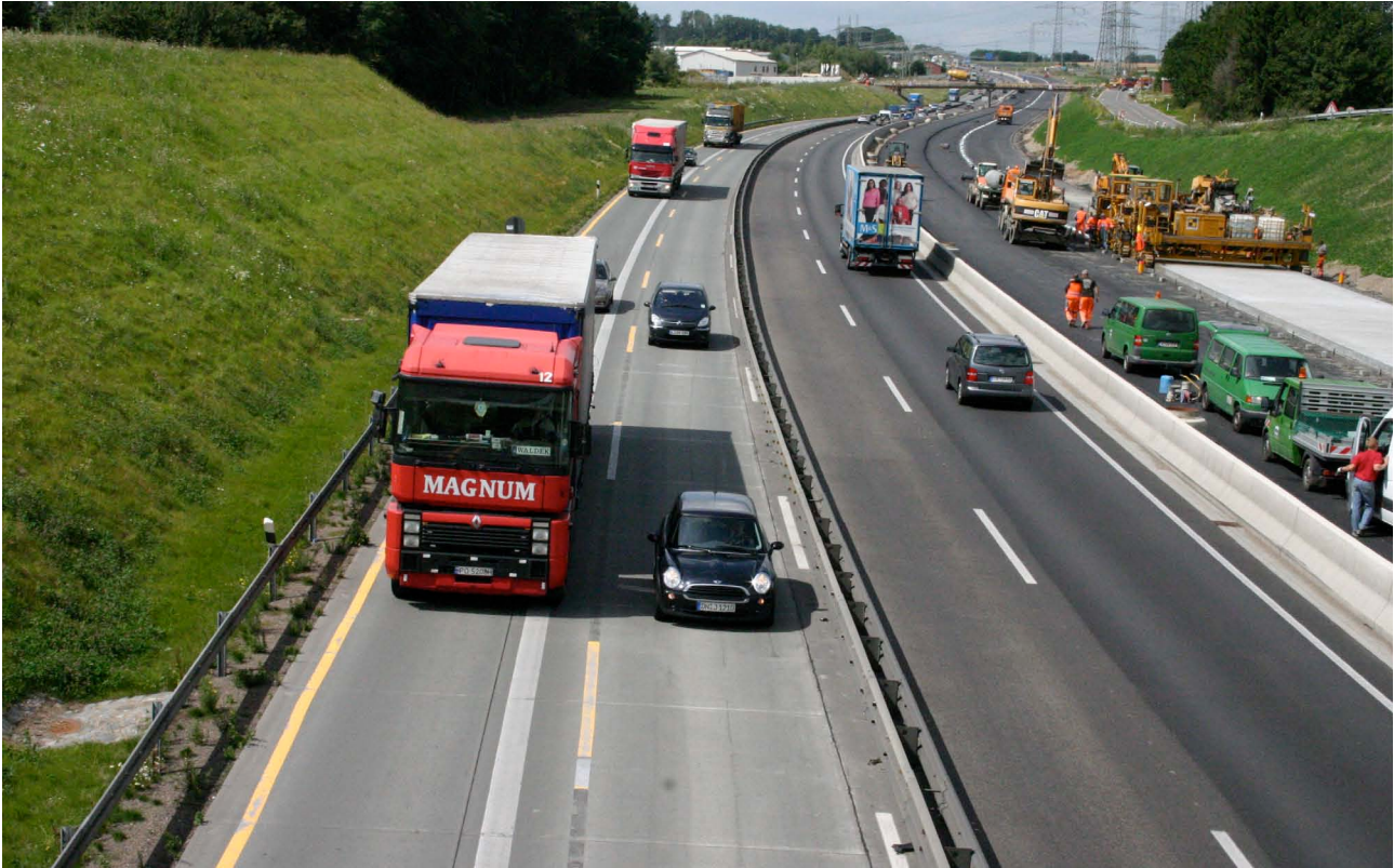
Construction site of road widening in Germany (Ref: 7 and 9)
